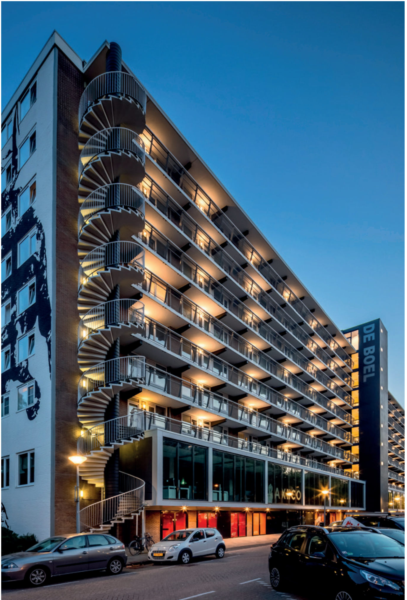
Apartment building De Boel - Amsterdam - Netherlands
