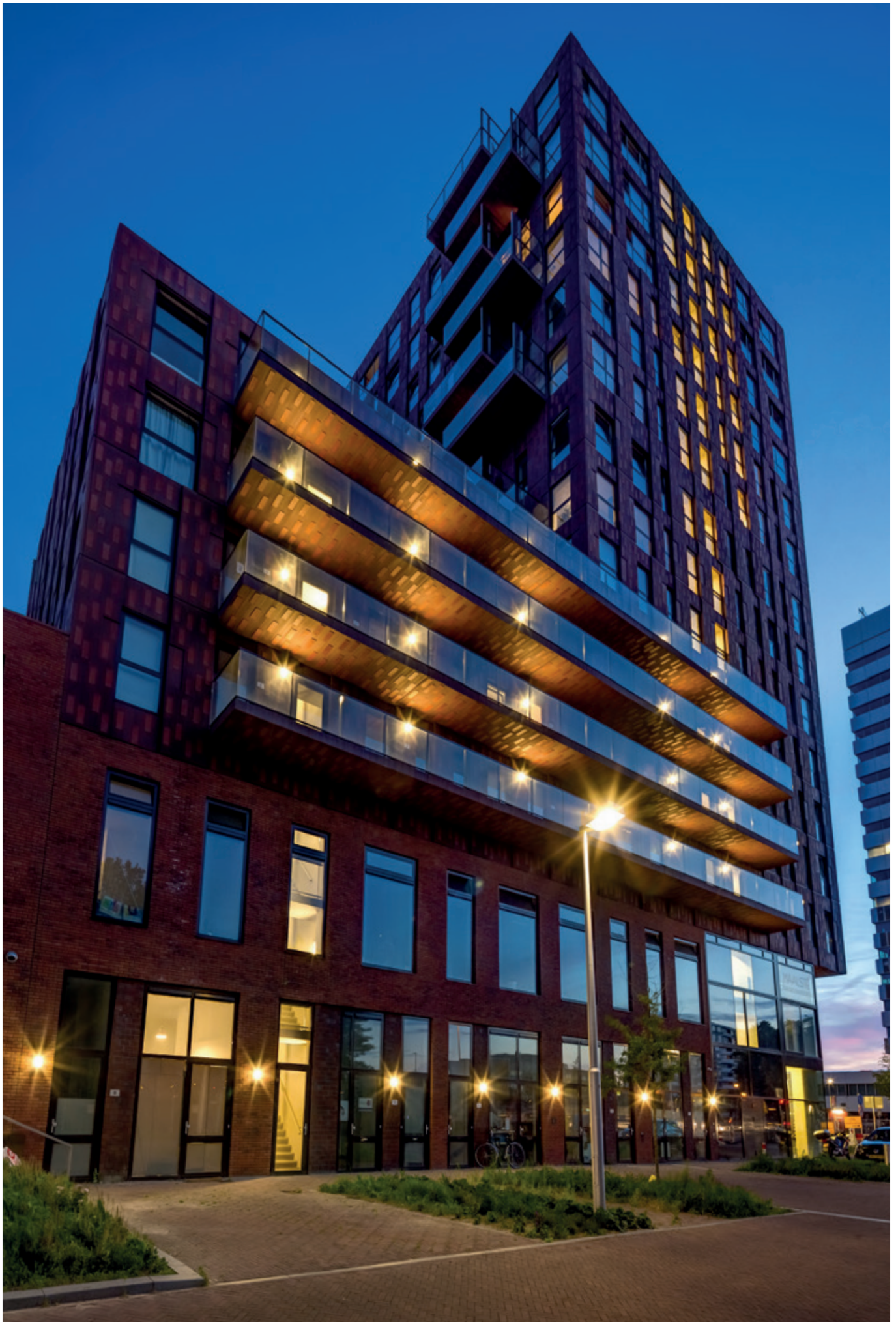
Residential Tower De Verkenner - Utrecht - Netherlands
