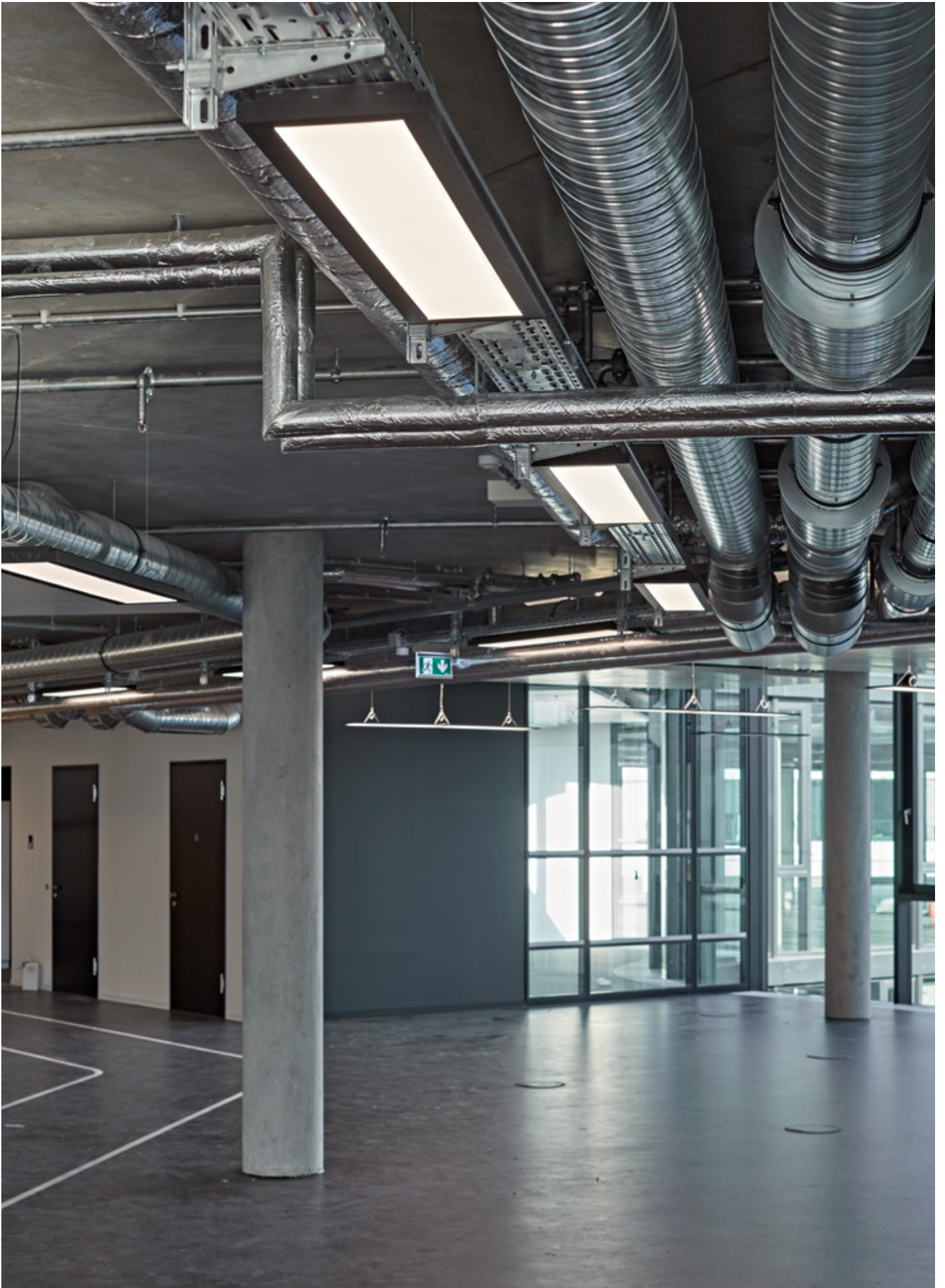
Zalando headquarters | Berlin | Germany
