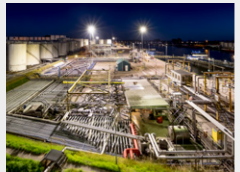
Tank storage Standic B.V. | Dordrecht | Netherlands
